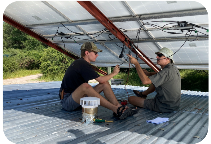
Aaron and Tim on the shed roof rewiring our solar panels.
